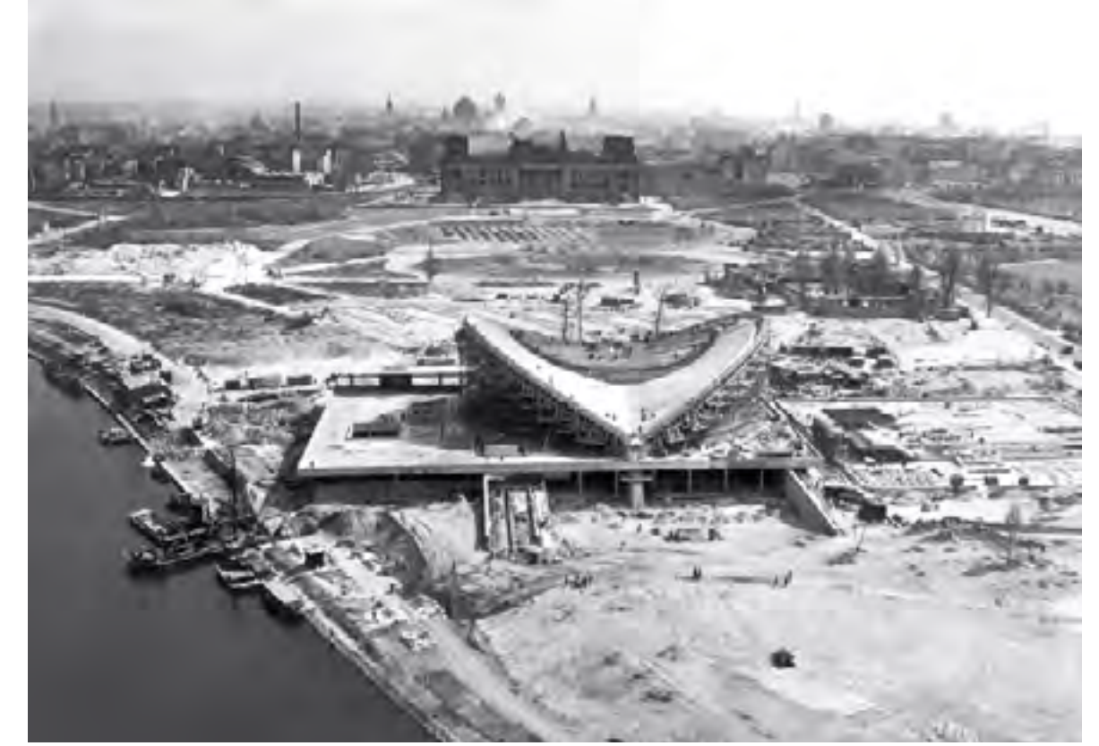
View of the Congress Hall under construction (as part of Interbau); the Reichstag building in the background, 1957
